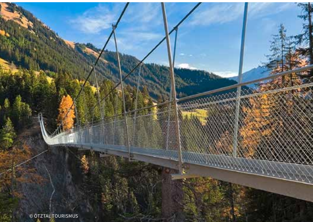
An 82 m steel structure across the Maurer Rinne near Längenfeld, at a height of 150 m.
